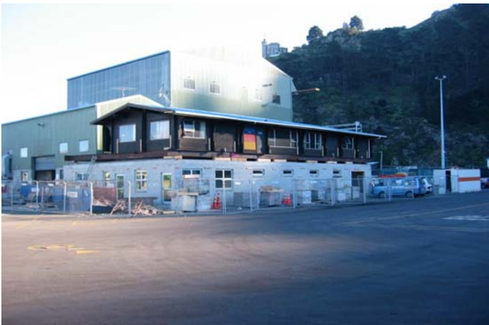
Sinclair Knight Merz designed a new understorey for an existing building for Lyttelton Port Company.
