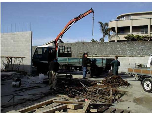
Recycling construction metal, Takapuna. (Avoca Construction)
