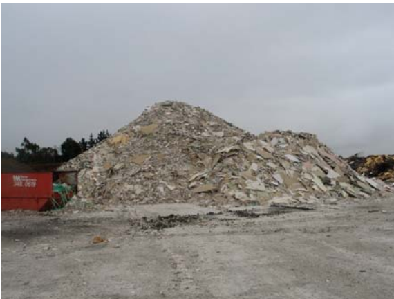
Plasterboard sorted from C&D waste, ready for processing, Crusaders Landscaping, Christchurch
